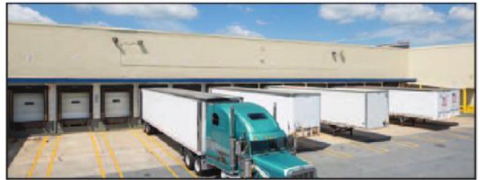
Rt. 61 Distribution Center
